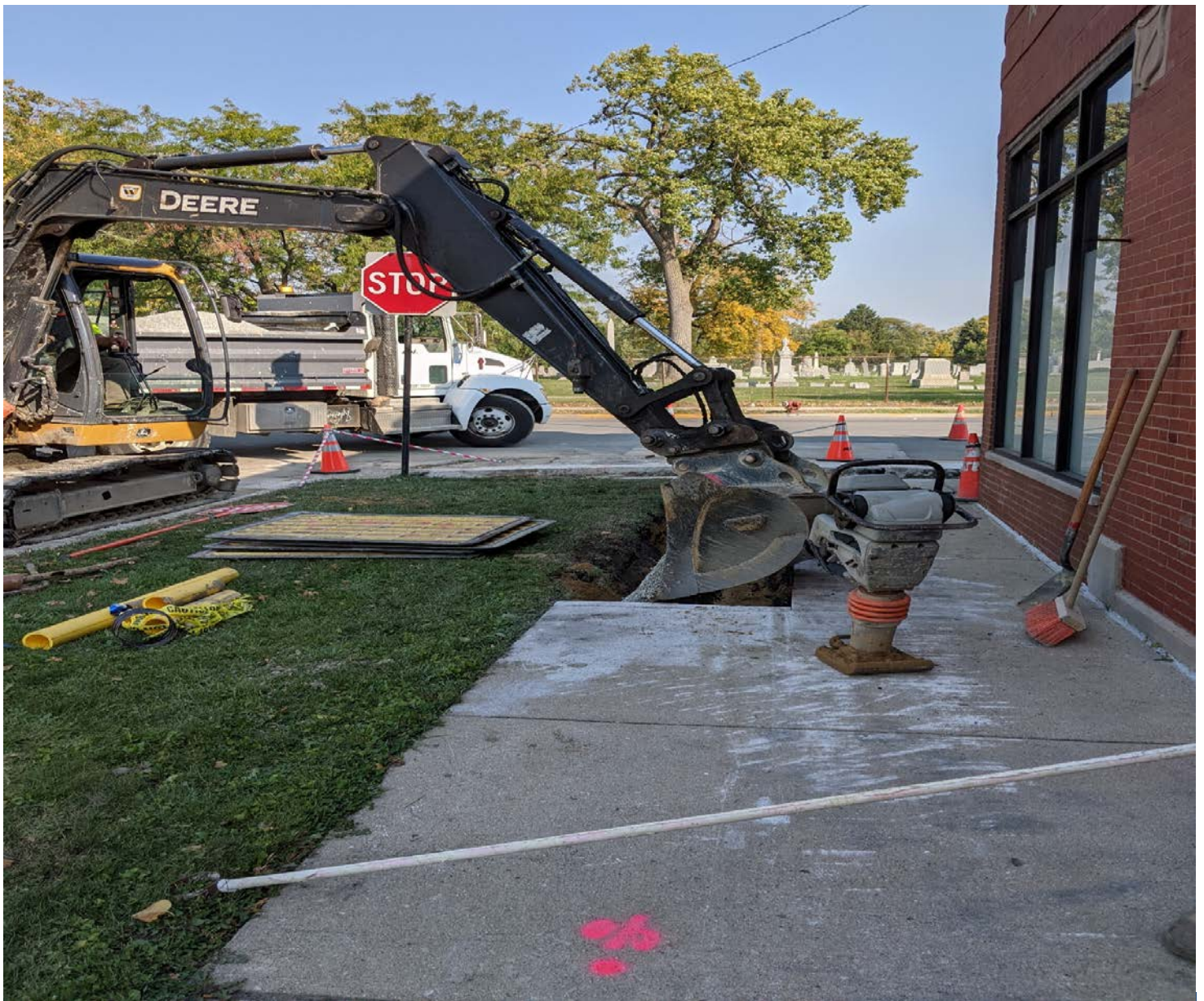
Schorsch Village Phase 1- Post valve installation on Nagle
